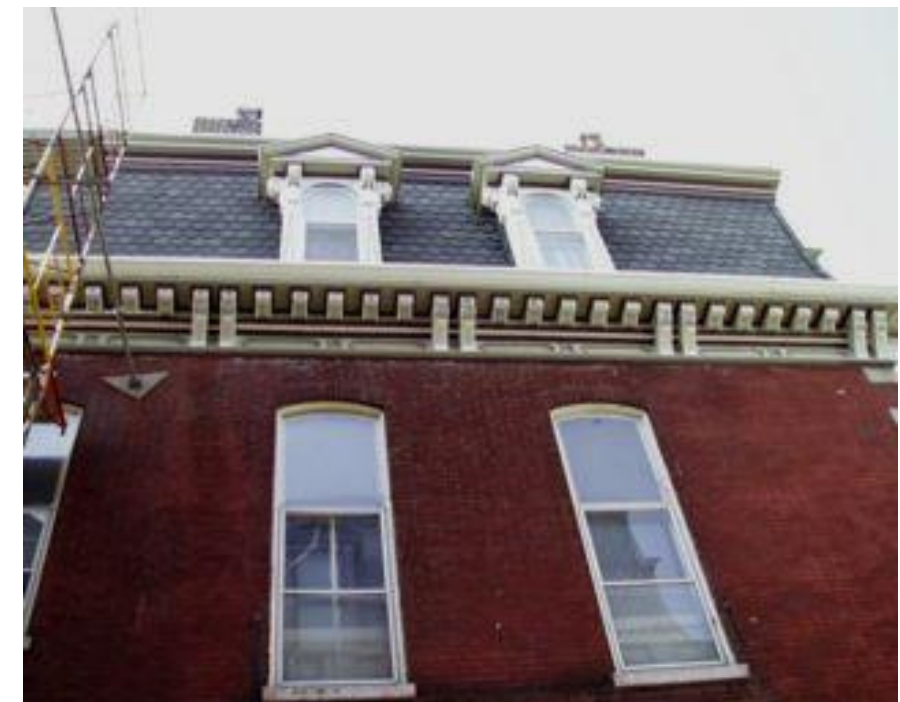
At right: an ornate cornice under a mansard roof with dentil molding
