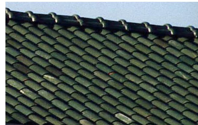
At right: a glazed clay tile roof
