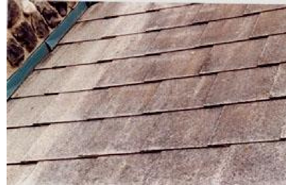
Above: side-lapped asbestos cement shingles
