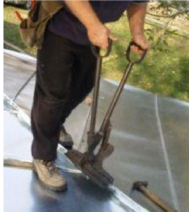
At left, An installer is crimping together the seams on a metal roof.
