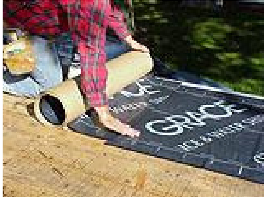
The lowest 3 feet of the roof get a layer of ice and water shield.
