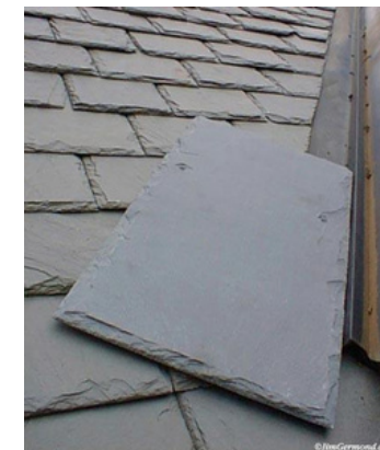
At right: a new slate roof; notice the crisp edges on the slate.
