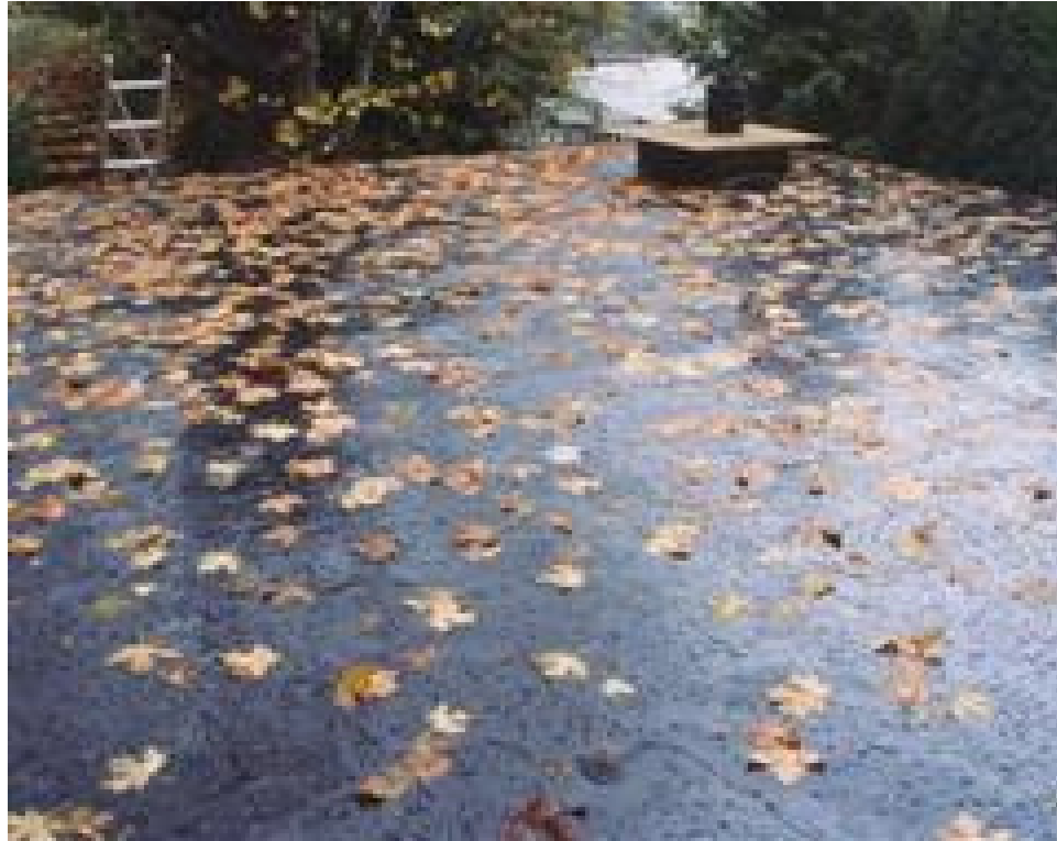
Above: This is a standard rubber membrane roof on a commercial property.
