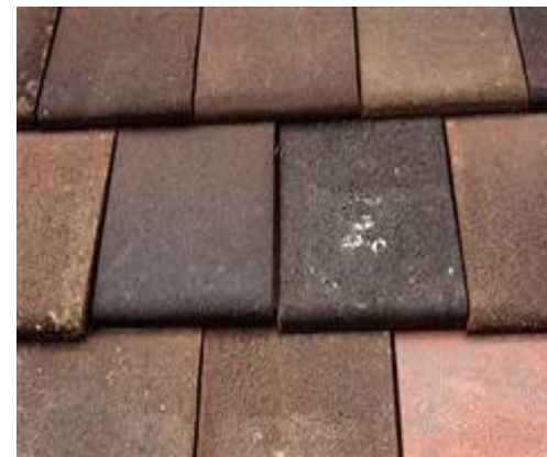
At left: a flat clay tile roof
